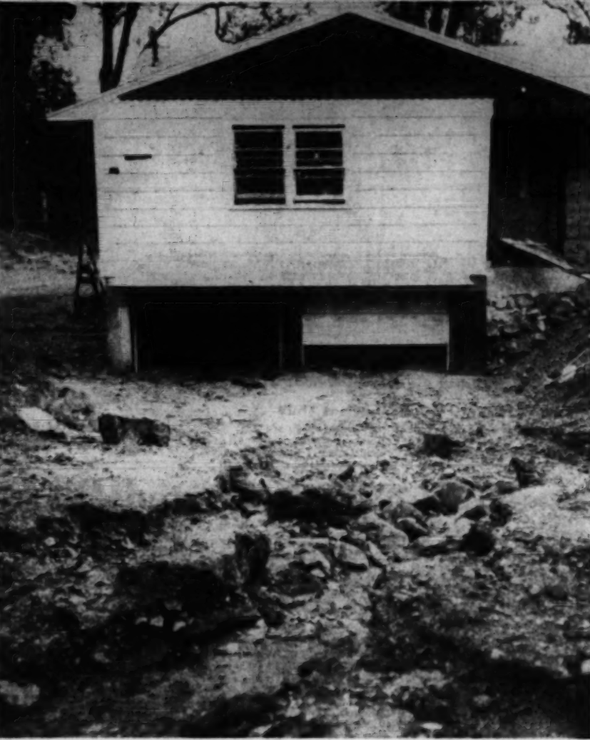
New England Digs Out From Diane's Downpour This home, under construction in Needham, Mass., was faced with new problem of excavation when mud and stones flowed into garage. All over New England relief work moved swiftly.
